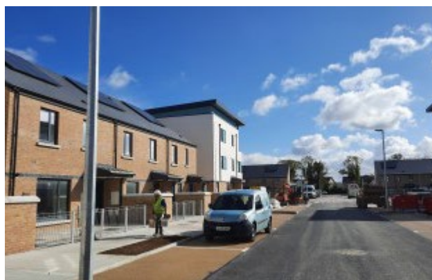
Completed housing development, Nancy's Lane in Clane, Co. Kildare
